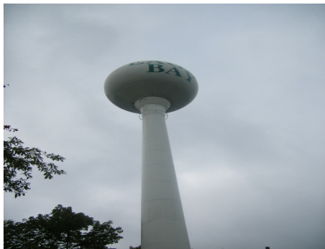
Figure 3: Phase 2 WiMAX antenna location
