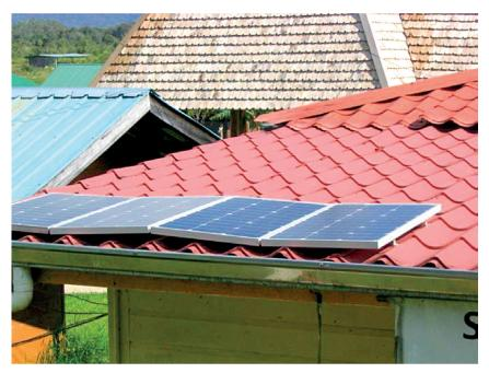
Figure 2-2-4: Solar panel installation on bario telecentre's rooftop
